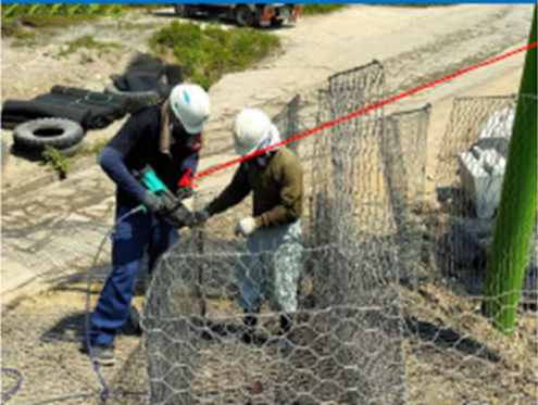
碎石投入状況と型枠
